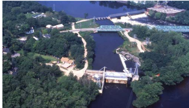
Bar Mills Dam (credit: FPLE)
